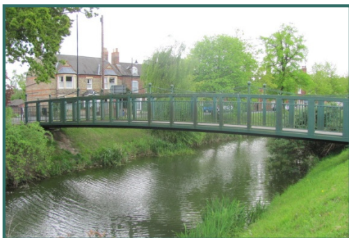
River Welland Footbridge
